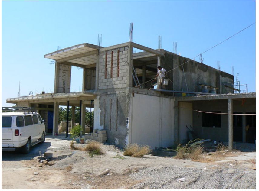
Above: Progress on Ministry Base
