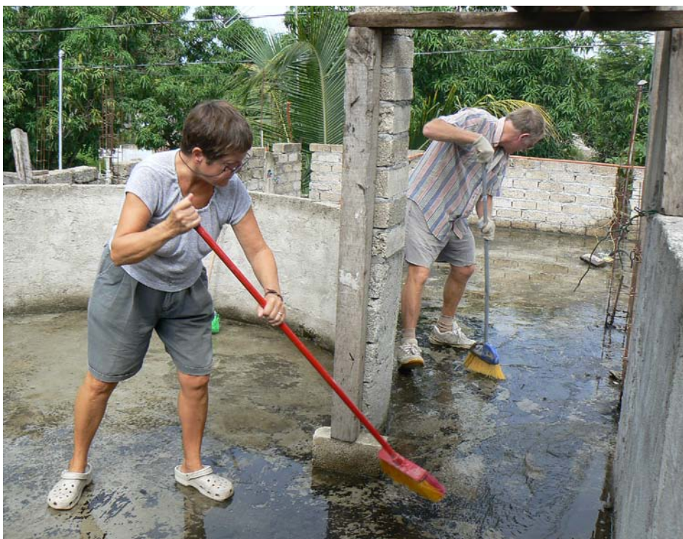
Madeleine & Alan Hanna preparing Carmen's roof for repair.
