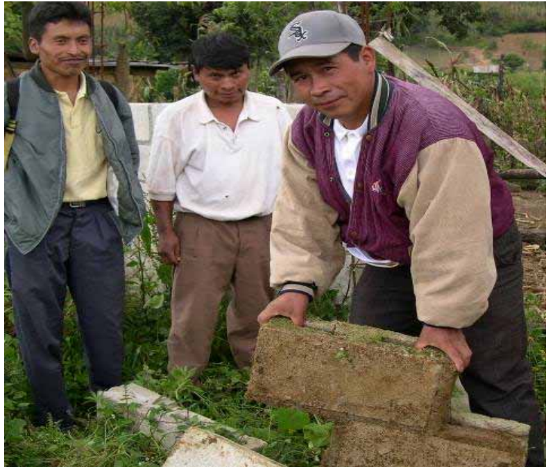
The walls and footings of this church severely damaged.
