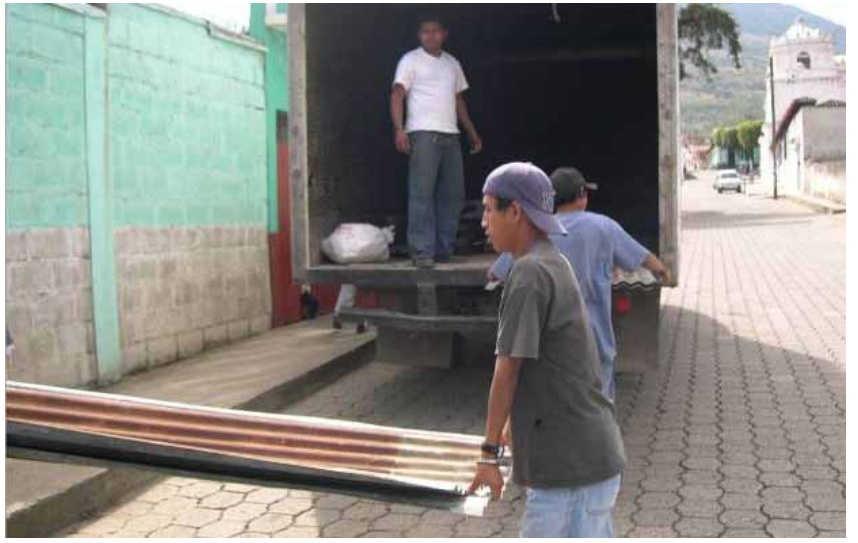
Youth assisting in the roof repair to the widow's home.
