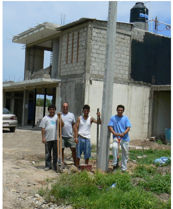
Everyone wanted to help dig the hole for the electric pole.
