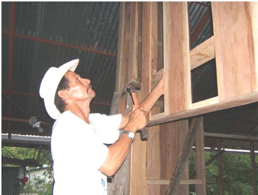
"Peek - A - Boo" walls under construction...
