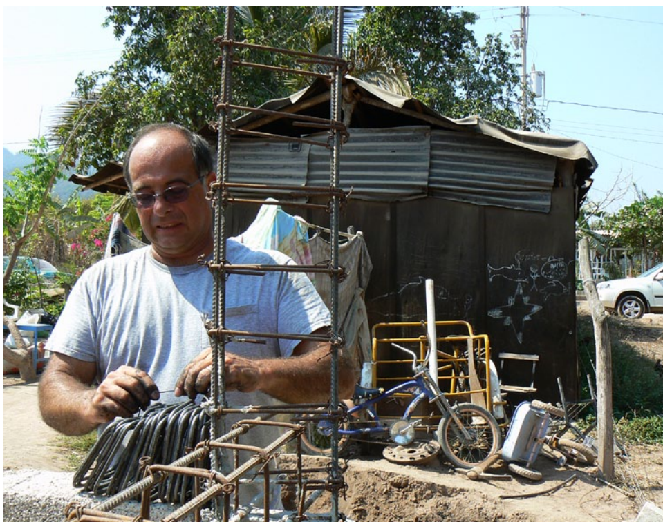
Lee works on the new construction behind the Ortega's present home.
