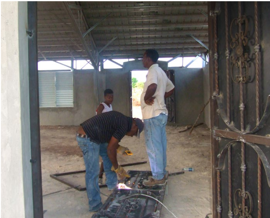
All field photos, church plant & children's center Dominican Republic
