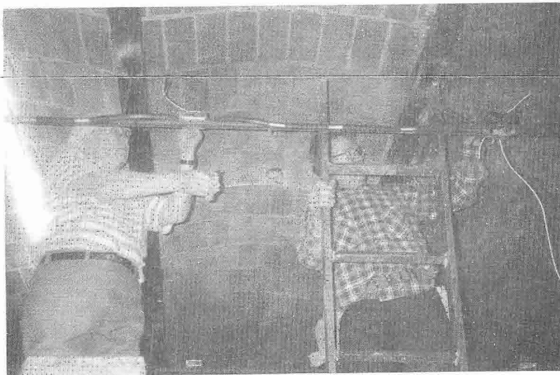
Milton and Frank wiring the studio light system.
