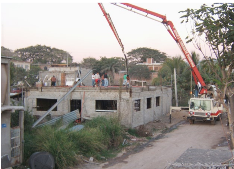
Pouring the roof for "Pan de Vida" at the Municipal Dump.
