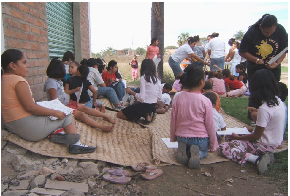
Kid's club moved outside due to construction preparation for the roof pouring.
