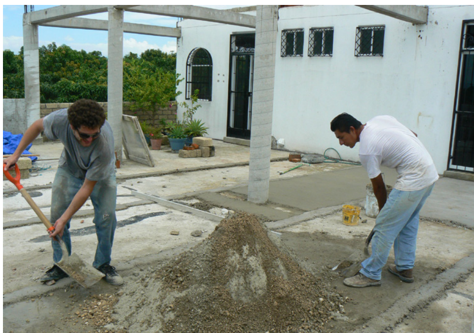
Eddie Hudson & Pastor Miguel sealing the roof over the Children's Center
