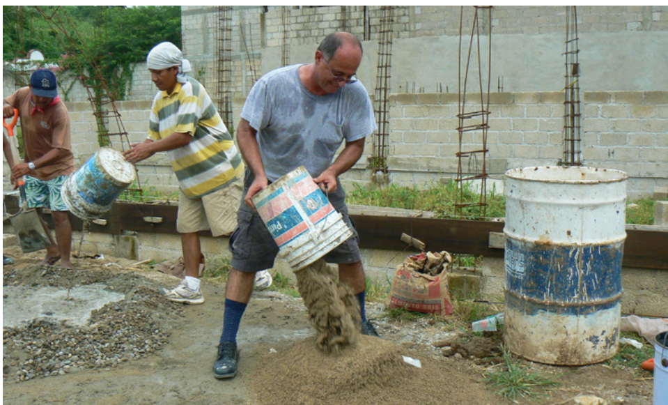
Lee & Jamil lending a hand with Ixtapa church construction
